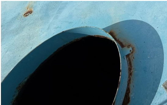
Heavy Corrosion on Bowl Access Hatch Curb
