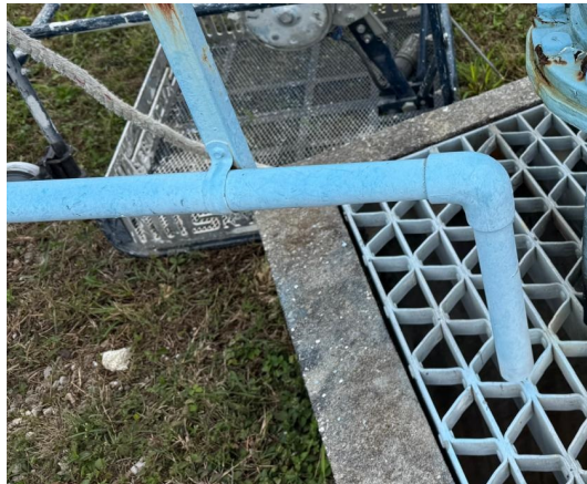
Condensation Drain Line
