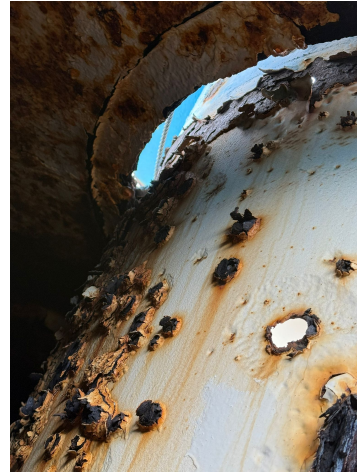
Center Access Tube Passive Bowl Vent Penetration
