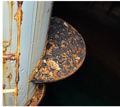
8-Inch Overflow Line Support Plate
