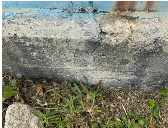
Vertical Crack in Concrete Foundation
