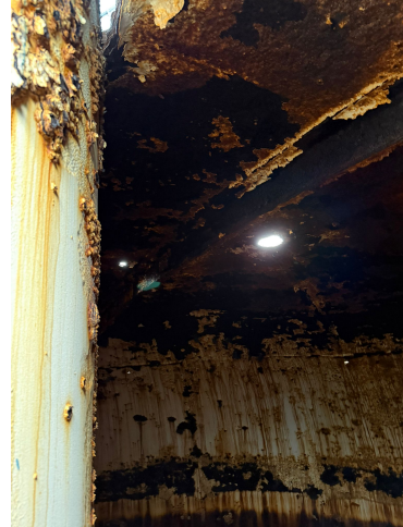
Severe Blistering Near Center Access Tube
