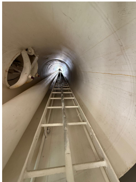
Pedestal Access Ladder and Safety Cable
